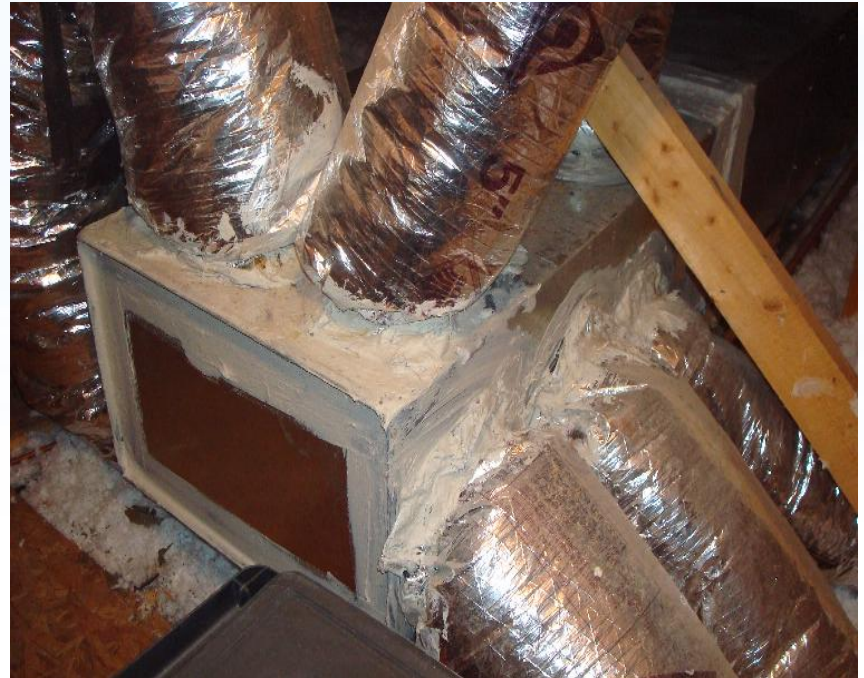
Joint and seams thoroughly sealed
